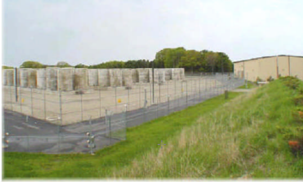
Figure 9. Dry cask storage of spent fuel. Two casks typically contain the equivalent of a year's spent fuel discharges from a 1000 MWe nuclear power plant. Comparison of the simplicity of interim spent fuel storage with the complexity of the huge reprocessing complex shown in Figure 6 makes it easier to understand the relatively low cost of interim storage. 17
